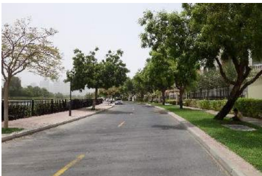
Corniche First Street, access to the Property
