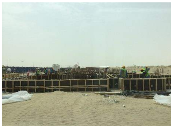
Foundation works for townhouses
