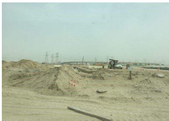
View of project
