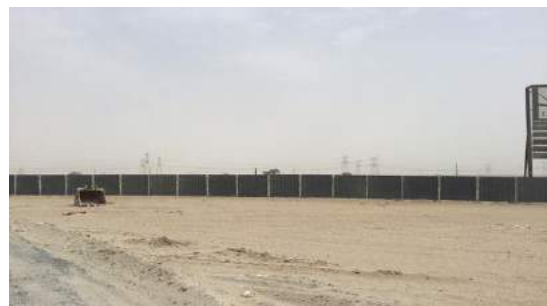
Boundary along internal road
