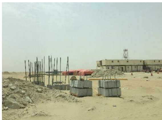
Preparations for construction works
