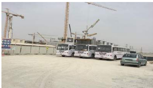
View of project under construction
