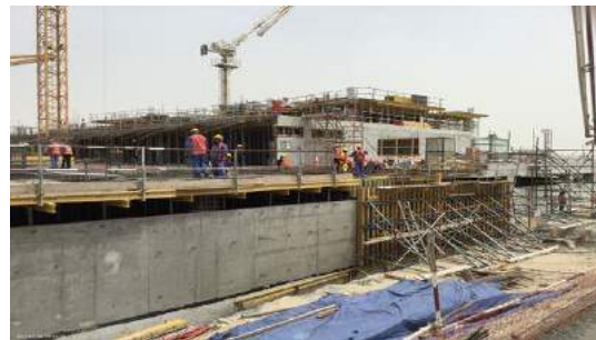
View of project looking north-east
