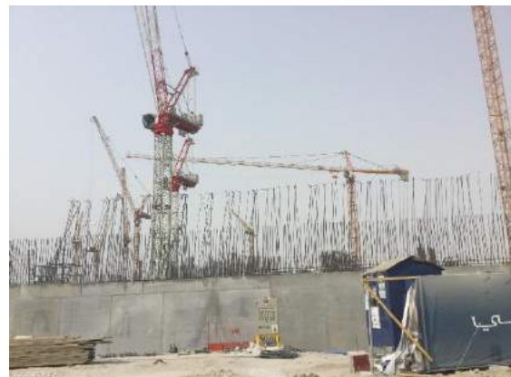
North View of Property
