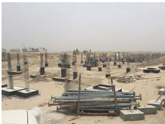
Fairway Vista construction
