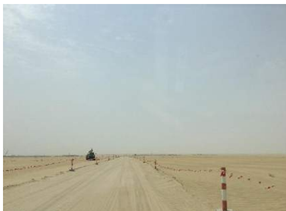
North easterly view of the Project
