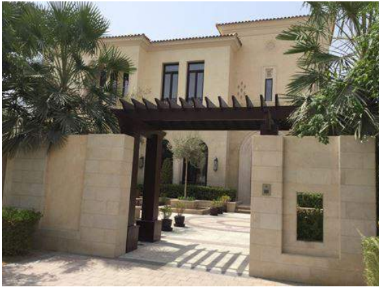
Unit SD – 17, entrance
