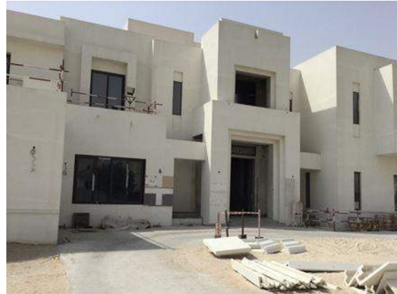
Unit SD – 18, external elevation
