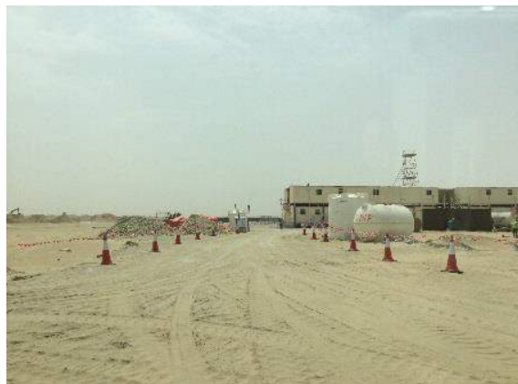
North easterly view from the boundary
