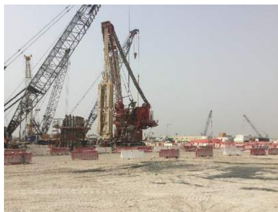
The Tower construction site
