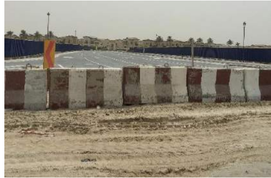
Plot PA04 – road (under construction) dividing PA03 and PA04
