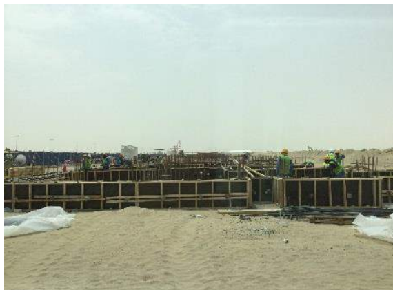
Foundation works for townhouses
