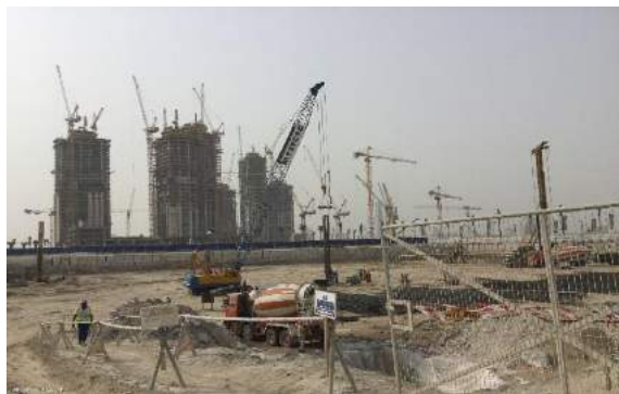
North view of Property
