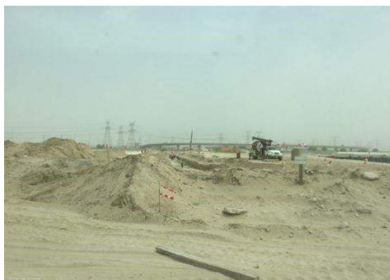
View of project
