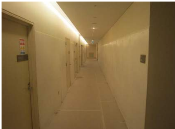
Typical internal corridor
