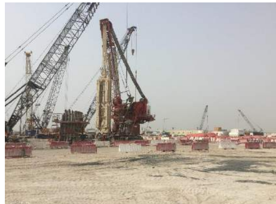
The Tower construction site
