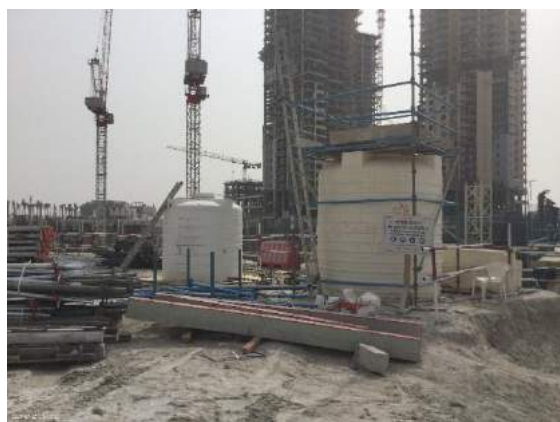
West View of Property
