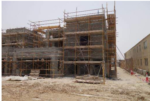
Villa under construction
