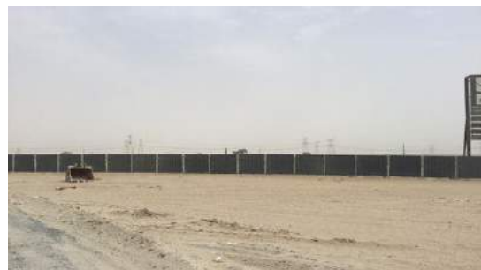
Boundary along internal road
