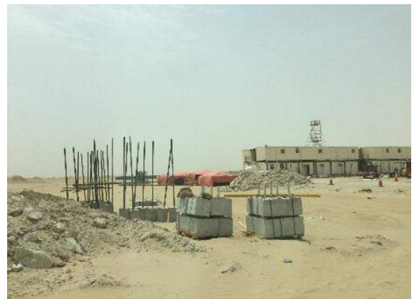
Preparations for construction works
