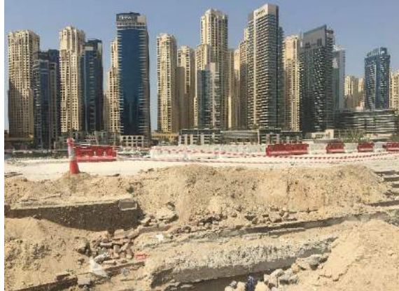
Northerly view from boundary
