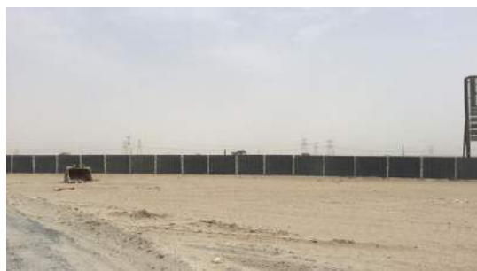
Boundary along internal road
