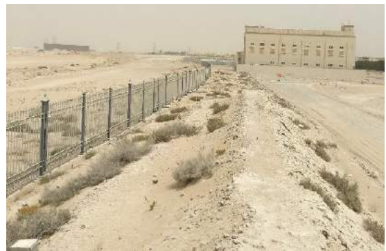
Plot PA03 - eastern boundary with DEWA substation
