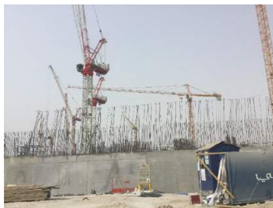
North View of Property
