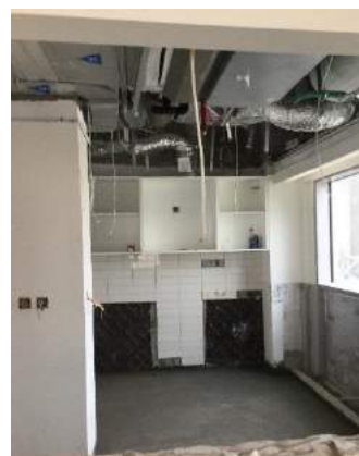
Under construction kitchen
