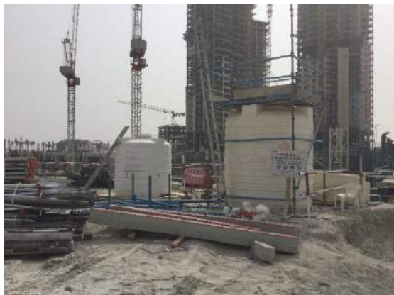
West View of Property
