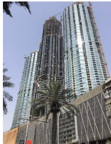
External view of façade
