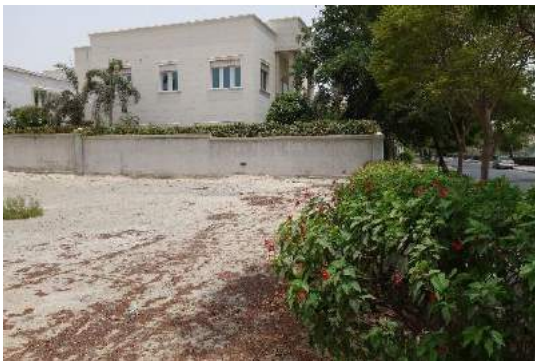
View from Corniche First Street
