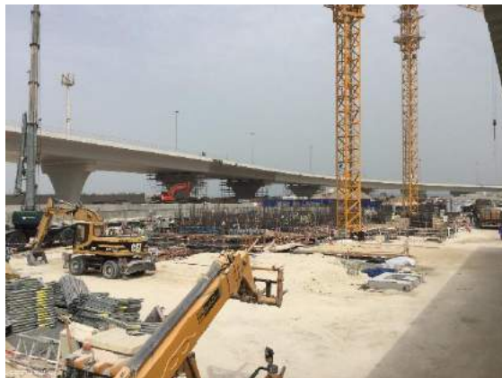
View from the east looking towards Tower 1
